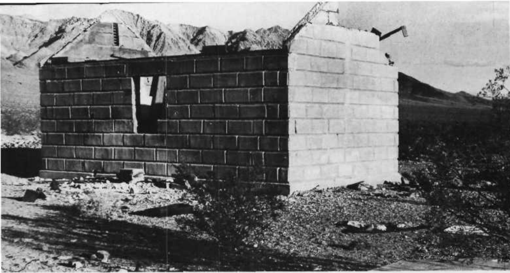
Large boulders of marble mark the entrance to the old railroad bed (left) which is now a steep road leading to the ghost town (above, left) of Carrara. Chandler machines (below, left) were used to cut the marble blocks. Edward
